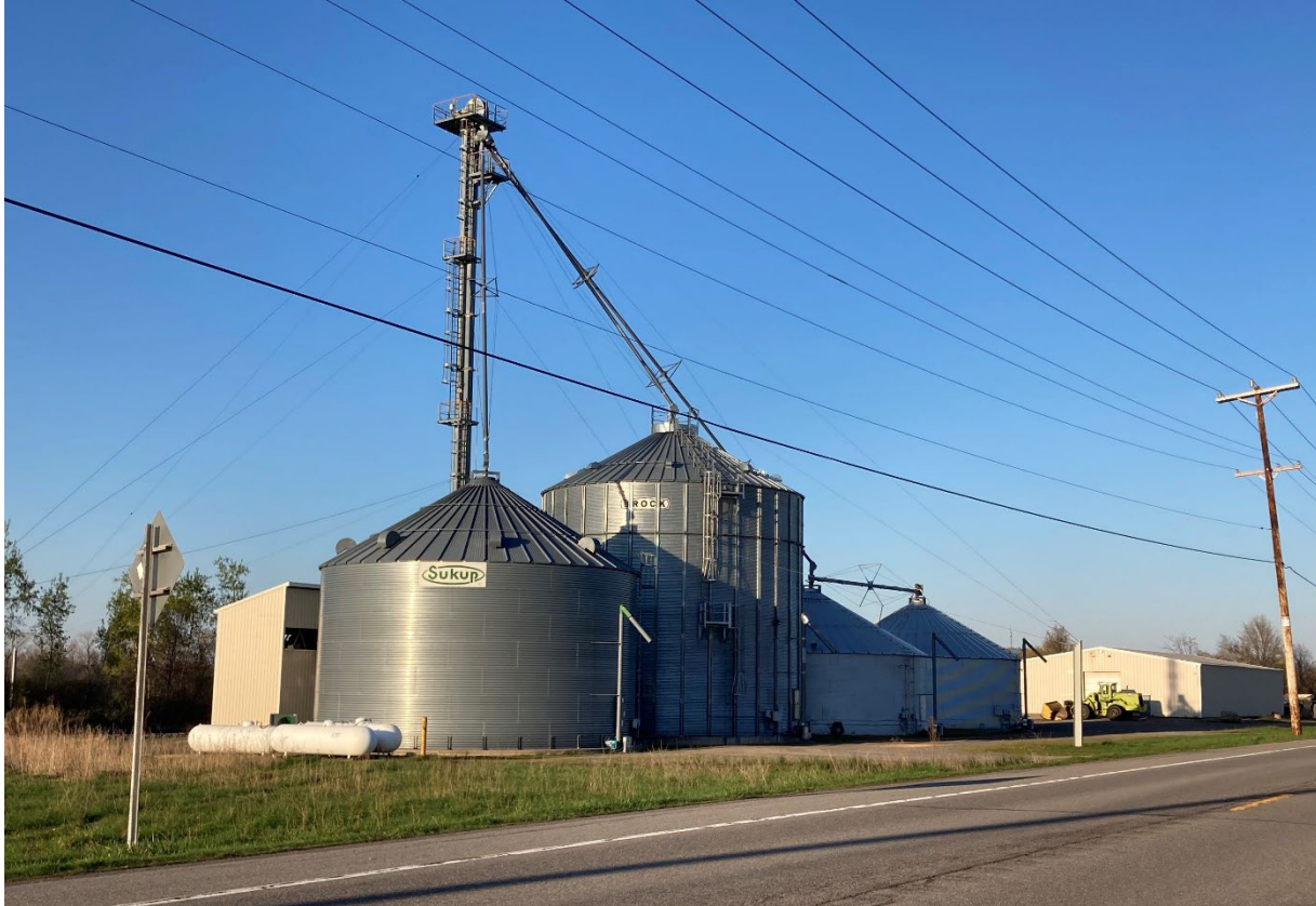
Figure 5 Storage tanks in Murray
